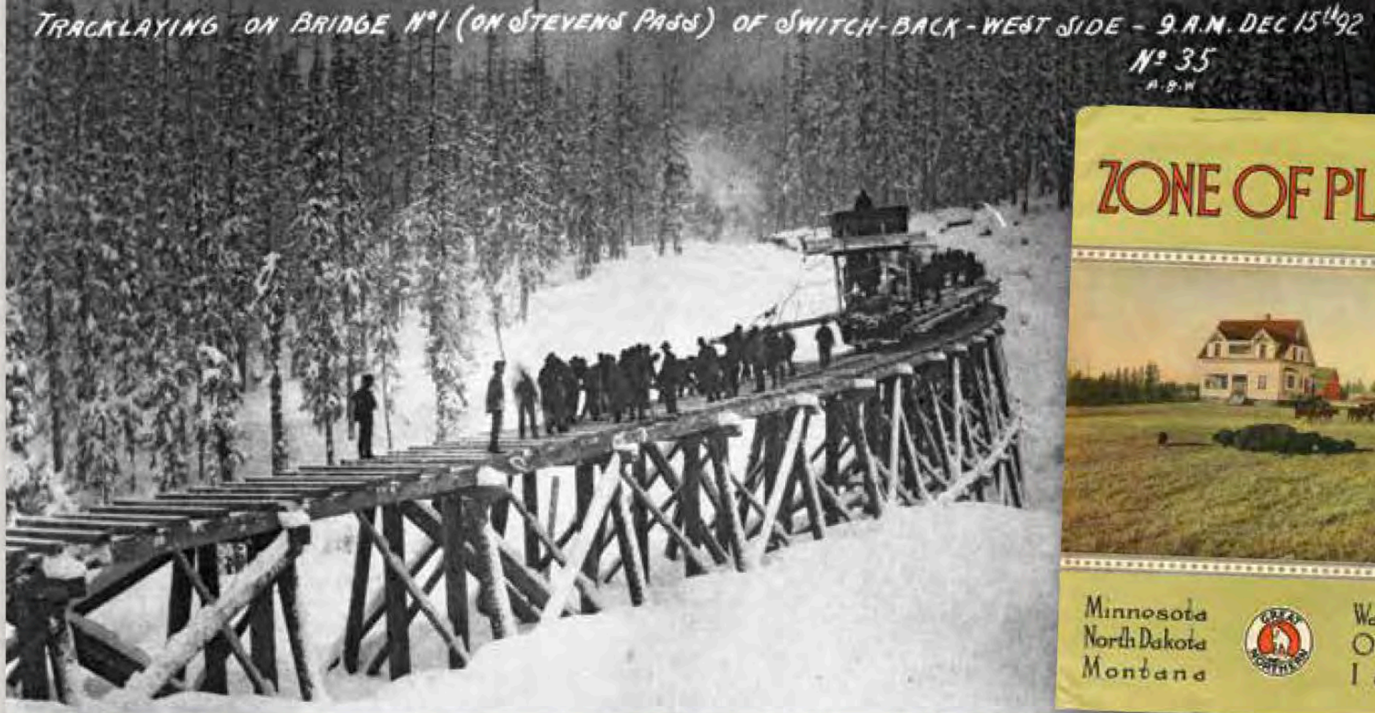
LEFT: Laying track on Bridge No. 1, Stevens Pass, switchback, west side, December 15, 1892. Construction of the Great Northern extension to Seattle slowed substantially due to the winter weather and steep terrain of the Cascades. Anders B. Wilse, photographer. Washington State Historical Society, ID 2013.0.184.23. RIGHT: Zone of Plenty booklet about industries and agriculture in each state along the Great Northern's route. Circa 1928. Washington State Historical Society, ID 1997.10.98.
