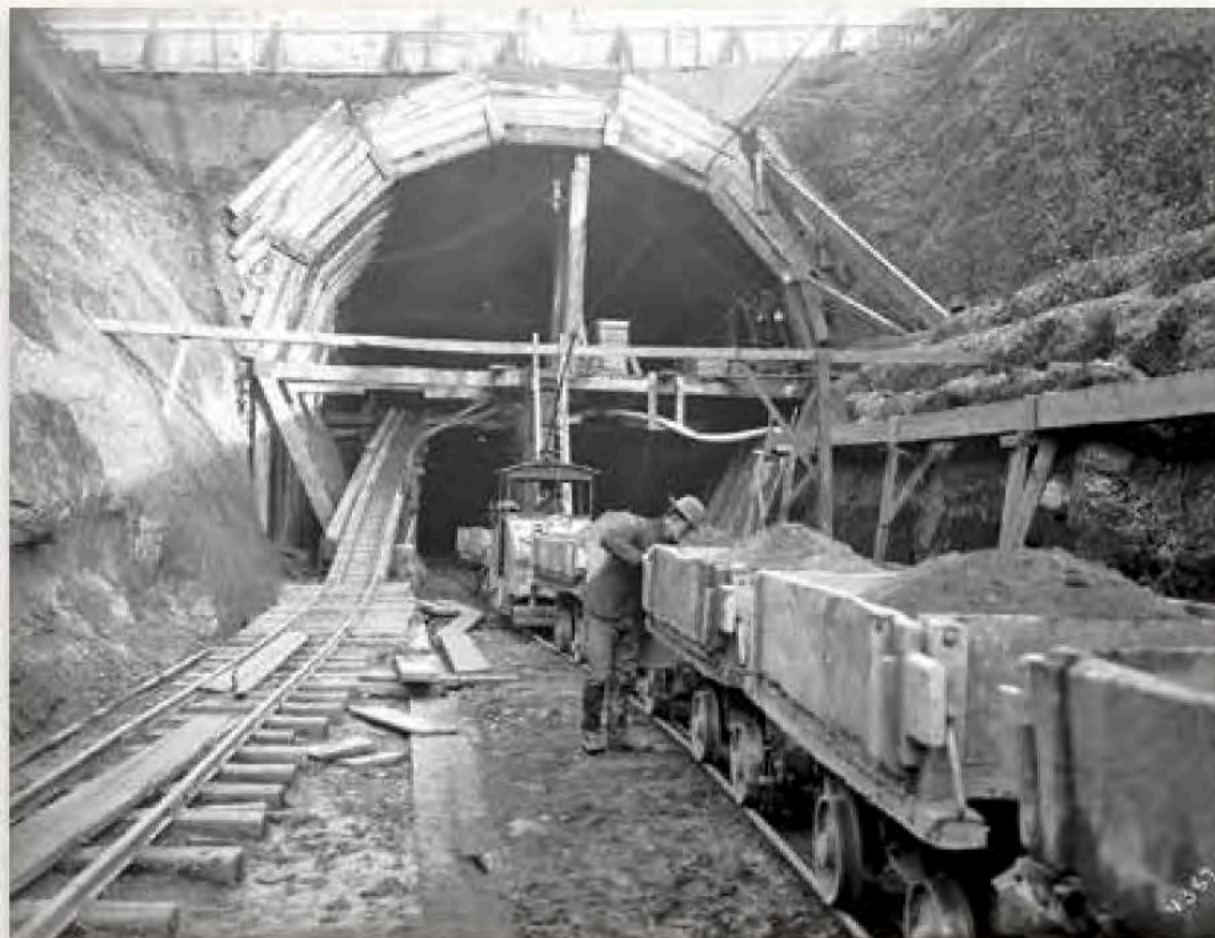
LEFT: Construction of the Great Northern tunnel under Seattle, January 19, 1904, built in partnership with Northern Pacific Railway, to prevent congestion downtown and provide access to the new King Street Station. The project employed 350 people. Small rail cars carried dirt from the excavation to fill in the tide flats at the southern end of the city. At a mile long, it was the highest and widest railway tunnel in the United States when it was completed and is still in use today. Asahel Curtis, photographer. Washington State Historical Society, ID 1943.42.4387. RIGHT: King Street Station Depot, Seattle, Washington, November 6, 1913. The station opened on May 10, 1906, and served Great Northern Railway and Northern Pacific Railway. By purchasing market shares, James Hill and J.P. Morgan had gained control of the Northern Pacific in 1895. Asahel Curtis, photographer. Washington State Historical Society, 1943.42.28444.
