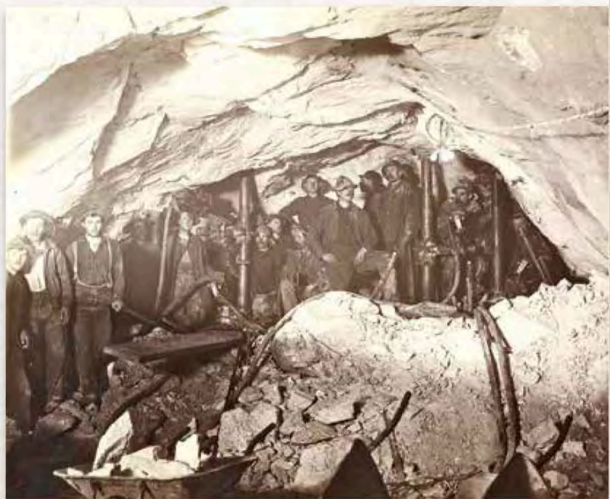
LEFT: Workers posing inside the Great Northern Railway Cascade Tunnel above Wellington, Washington, circa 1898–1899. Construction tools including metal braces, hoses for pneumatic drills, and a wheelbarrow are visible. When it was completed in 1900, it was the longest tunnel in the world, and another engineering triumph directed by John Stevens. Washington State Historical Society, ID 2010.185.4612B. RIGHT: Postcard of the entrance to Great Northern’s Cascade Tunnel, 1900. Courtesy Stephen Sadis. BELOW: Driving the last spike connecting the Great Northern Railway from Seattle in the west to St. Paul in the east. Scenic, Washington, January 6, 1893. Courtesy Minnesota Historical Society, YR1956.7896.
