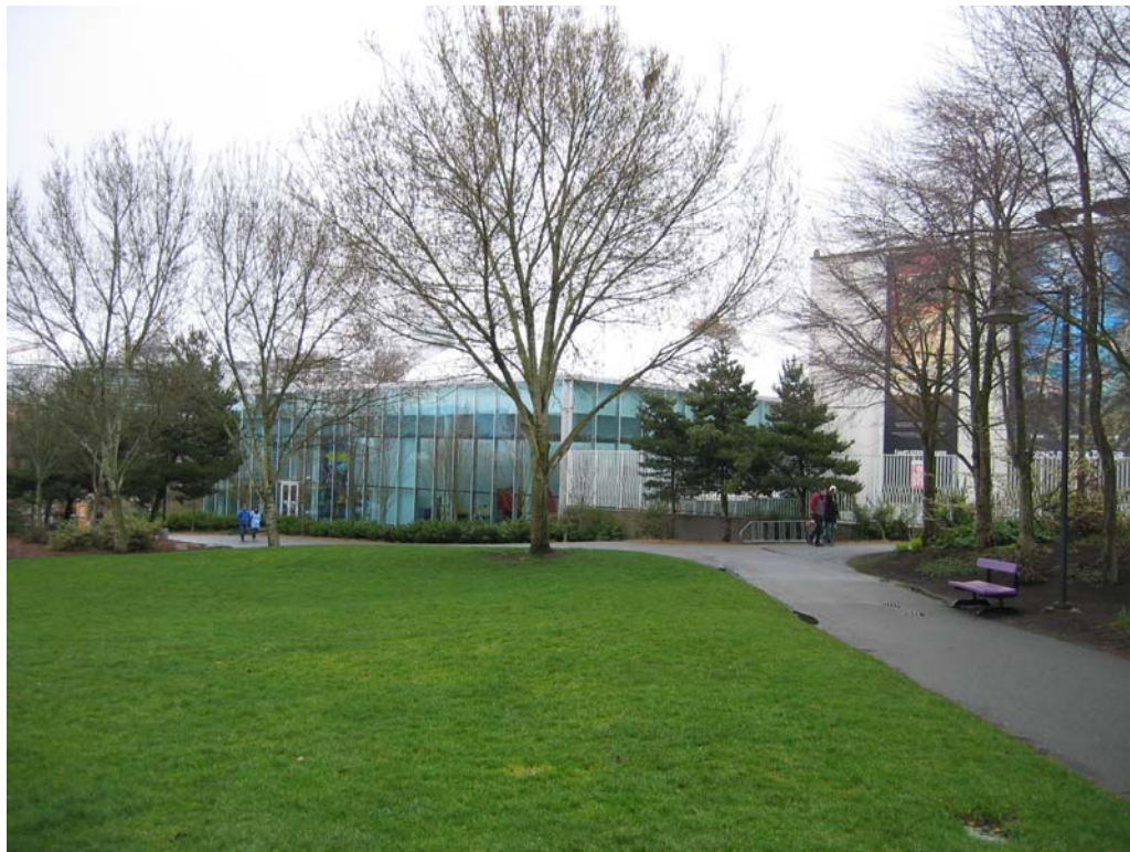
Figure 41 – Pacific Science Center, north elevation showing Building 1 (1962: Building 1) on right, and 1998 Boeing IMAX addition on left; view from Seattle Center grounds
