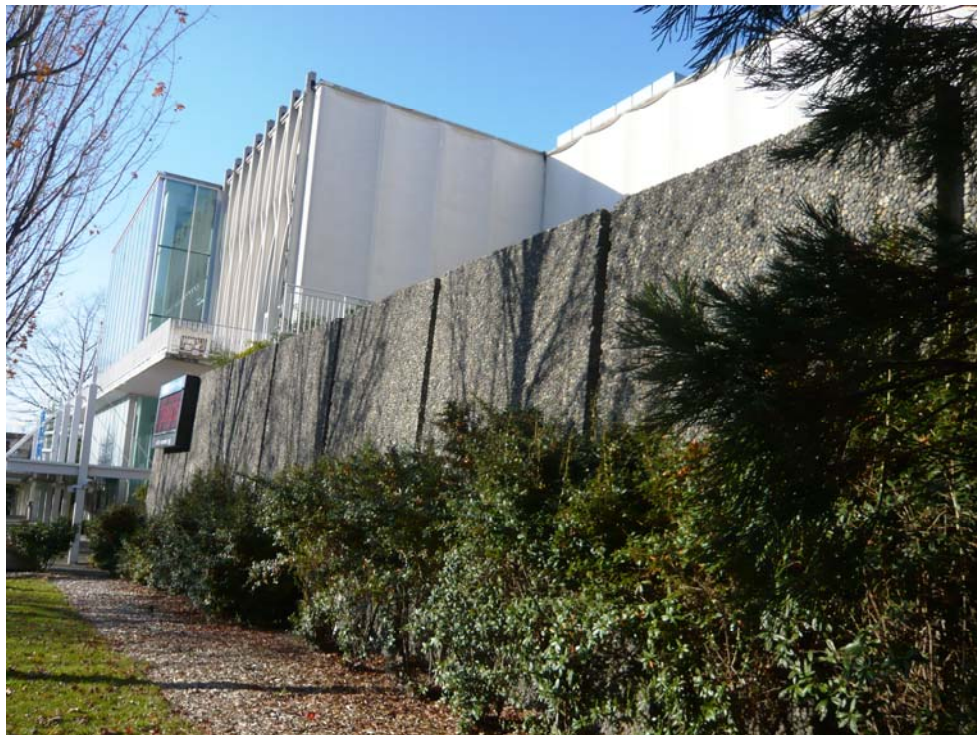
Figure 91 – Southeast Terrace pebbled retaining walls in foreground; south and east elevations of Building 3 (1962: Building R) at upper left; south elevation of Building 2 (1962: Building 4) at upper right.
