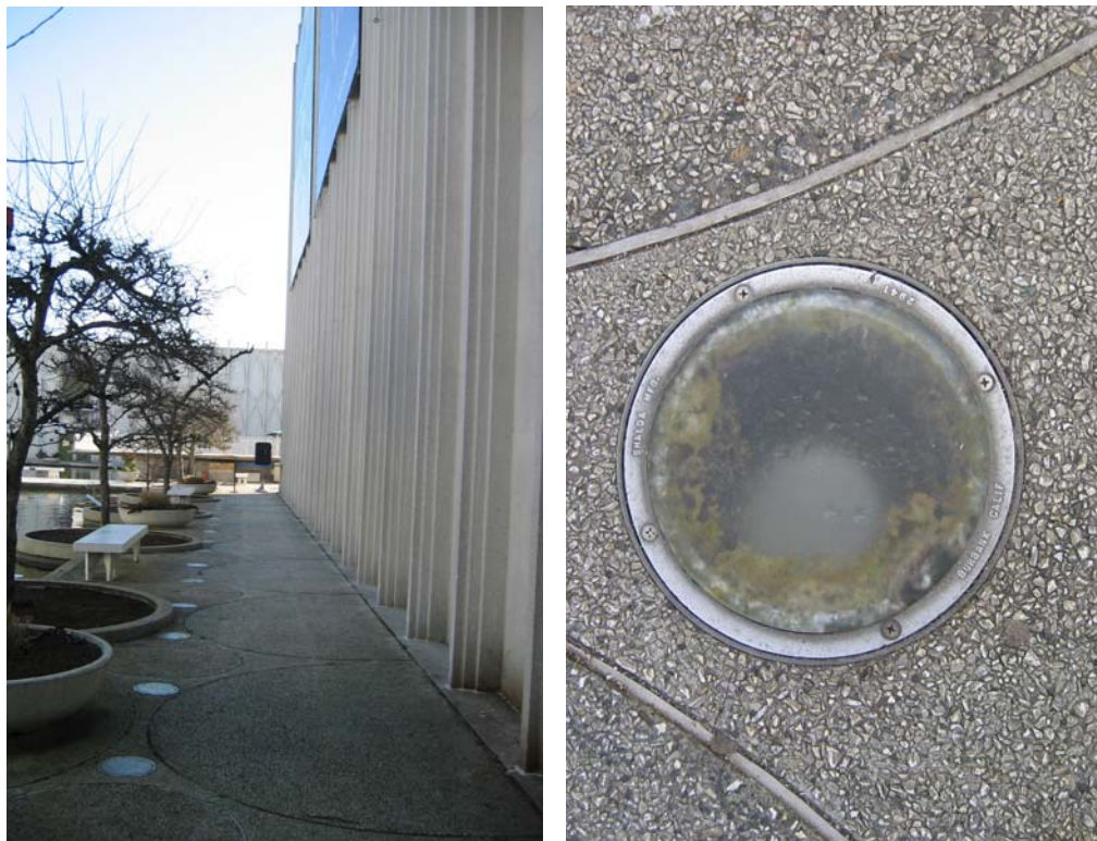
Figure 73 – 1962 recessed light fixtures in walks
