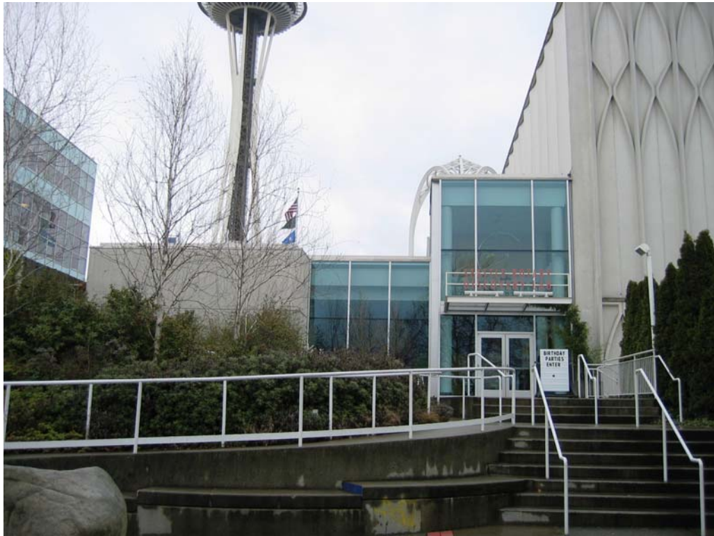
Figure 44 – Building 5 (1962: Building 1) on right, 1996 Discovery Labs addition on left (west elevation)
