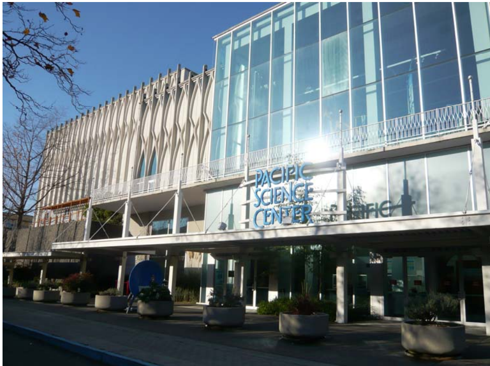
Figure 87 – South elevation of Building 4, Laser Dome, and Building 3 (left to right). The steel walkway canopy structure and large glazed bay dates to 1992-93 renovations to Building 3 (1962: Building R) to create a south entry at Denny Way. Railing and balcony at middle of picture is original to 1962 building.
