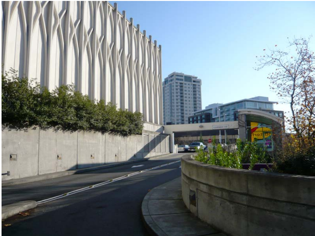
Figure 82 – West elevation, Building 4 (1962: Building 2), showing garage entry and drive aisle
