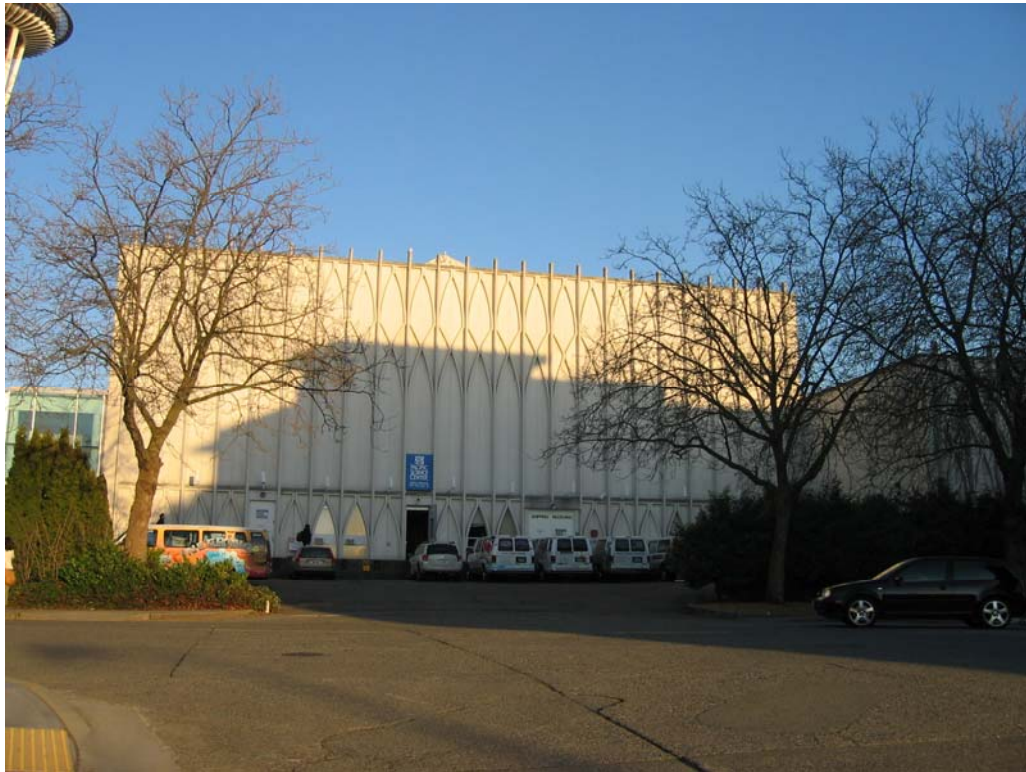
Figure 36 – Building 5 (1962: Building 1) west elevation, and loading dock
