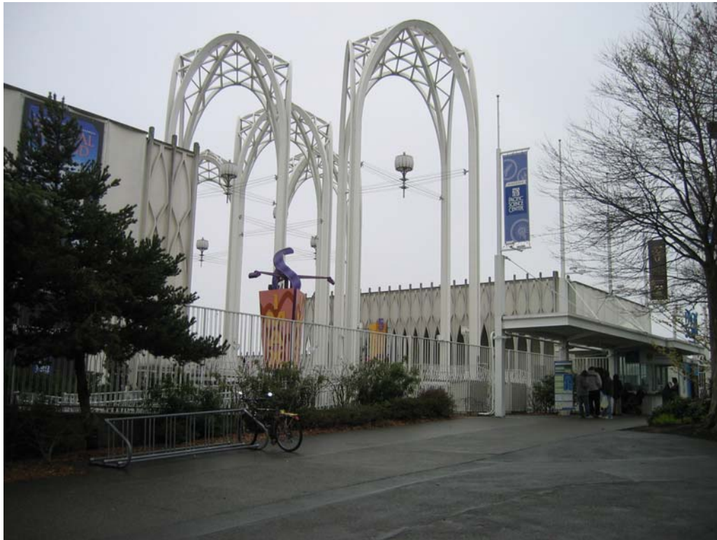
Figure 28 – North entrance forecourt and entry towers, from northeast
