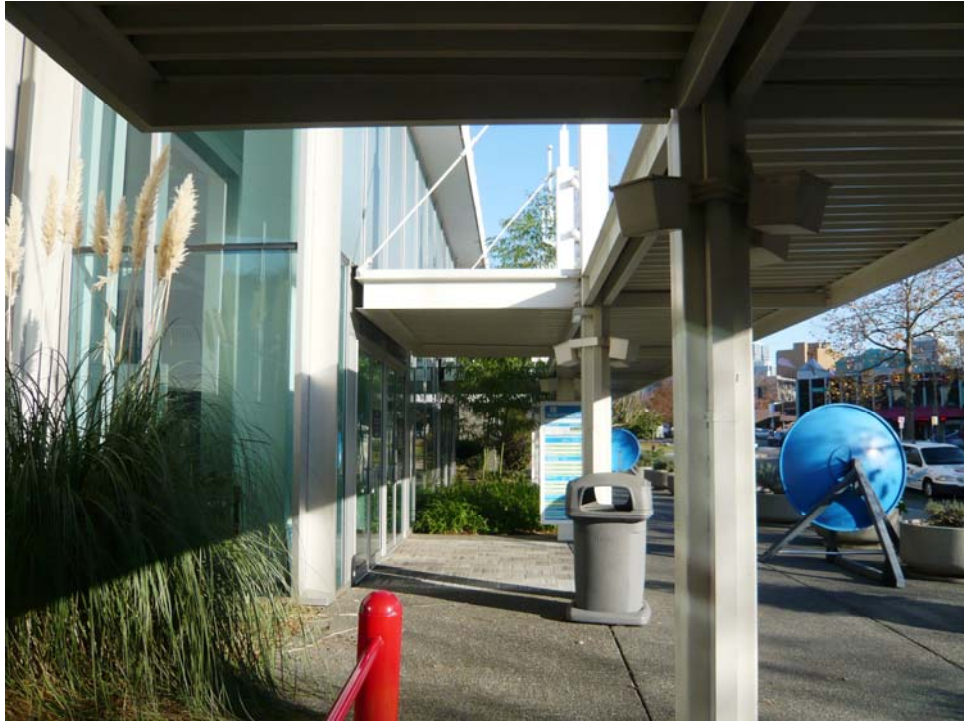
Figure 86 – Detail, south elevation Building 3 (1962: Building R). The steel walkway canopy structure dates to 1992-93 renovations to create a south entry at Denny Way.
