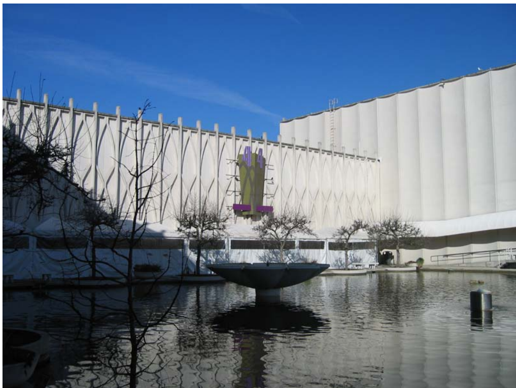
Figure 31 – Building 4 (1962: Building 2) east elevation, on left
