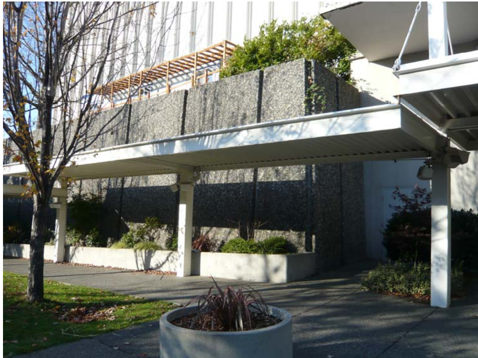
Figure 85 – South elevation of Laser Dome (1962: Building 3) in background, with south retaining wall of Southwest Terrace in foreground. A temporary office trailer is visible under a wood canopy. The steel walkway canopy structure dates to 1992-93 renovations to create a south entry at Denny Way.
