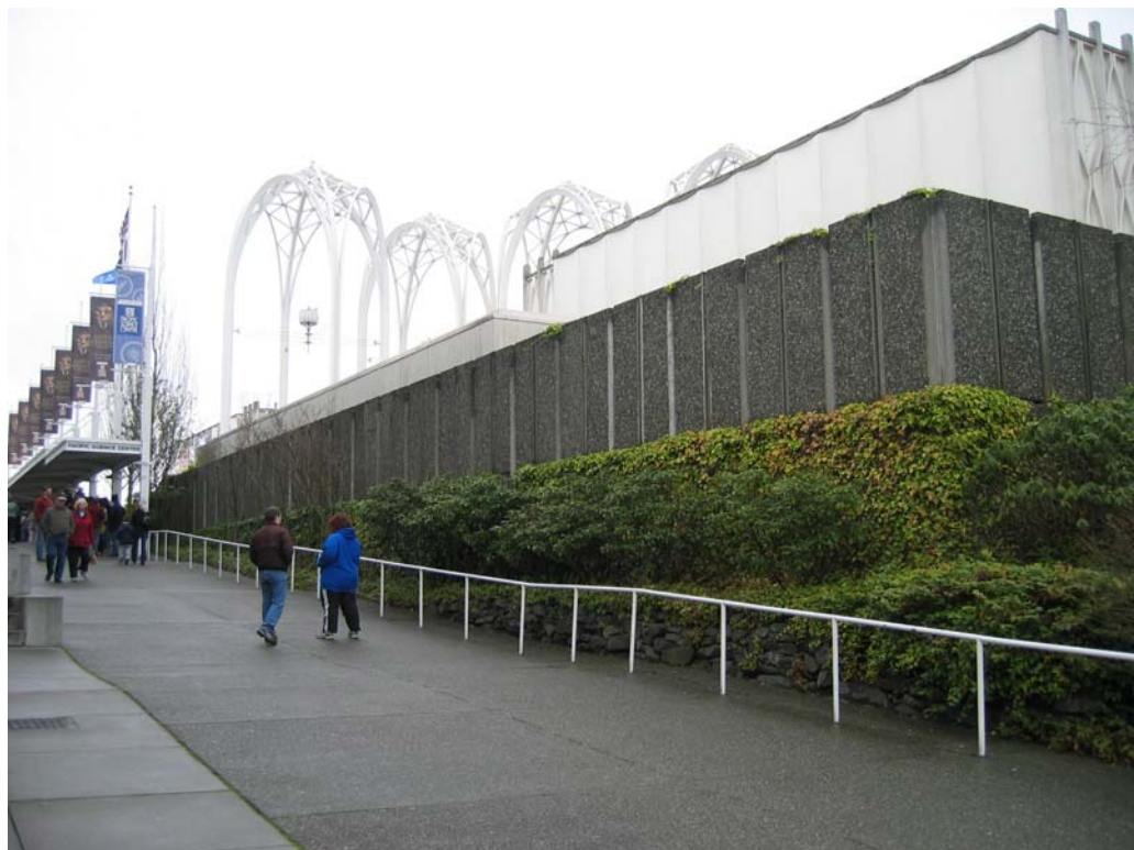
Figure 79 – Wall from 1962 West Exhibit Garden
