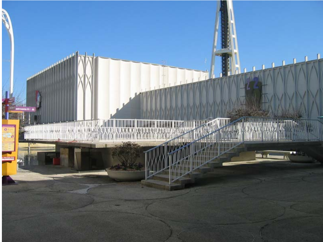
Figure 92 – Detail, Raised viewing platform at south end of Central Courtyard. West and south elevation of Building 1 at upper left, and west elevation of Building 2 at upper right. Base of the Space Needle is visible in center distance.
