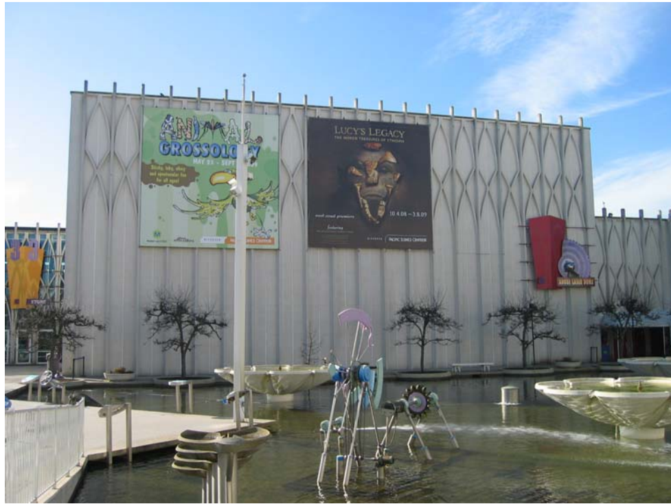
Figure 32 – Laser Dome (1962: Building 3), north elevation
