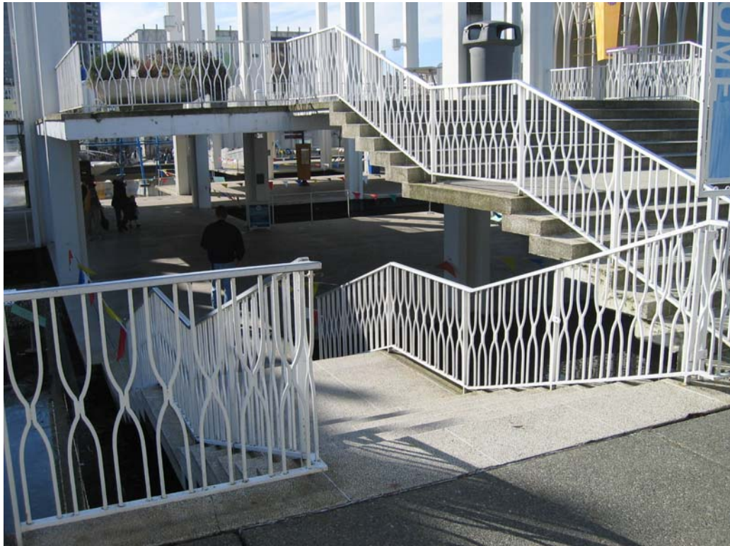
Figure 76 – 1962 stairs and railings
