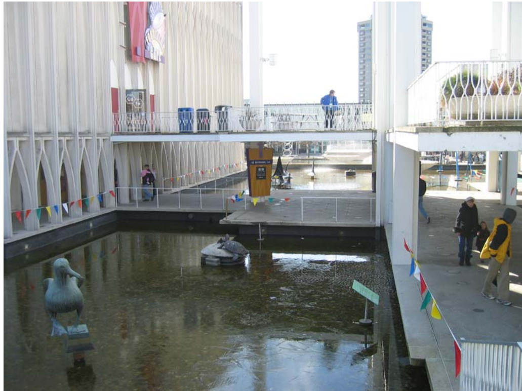
Figure 74 – 1962 walkways and railings
