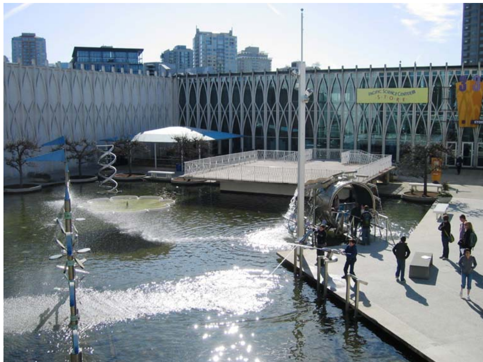
Figure 33 – Building 3 (1962: Building R), north elevation, on right; Building 2 (1964: Building 4) on left. 1962 viewing platform at center. Non-original features shown include 1993 pool pad and walk visible at right, tent, signage, glazed wall on Building 3, and all water features other than petalled fountain.
