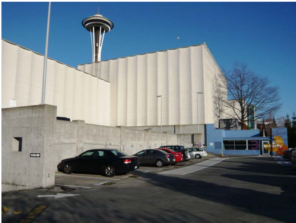
Figure 83 – South elevation Building 4 (1962: Building 2) at left; west and south elevation Laser Dome (1962: Building 3) at middle and right; view from Pacific Science Center Parking Garage (not on site).
