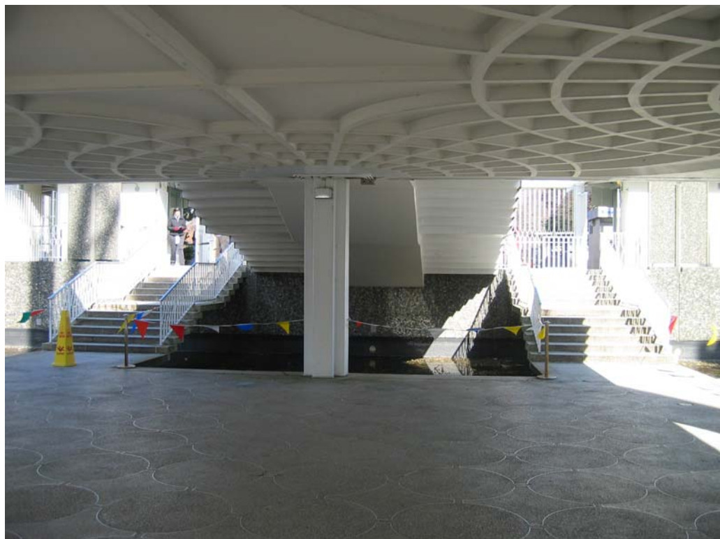
Figure 75 – 1962 underside of tower platform
