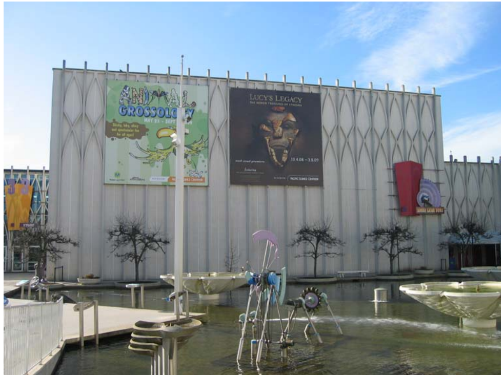
Figure 32 – Laser Dome (1962: Building 3), north elevation
