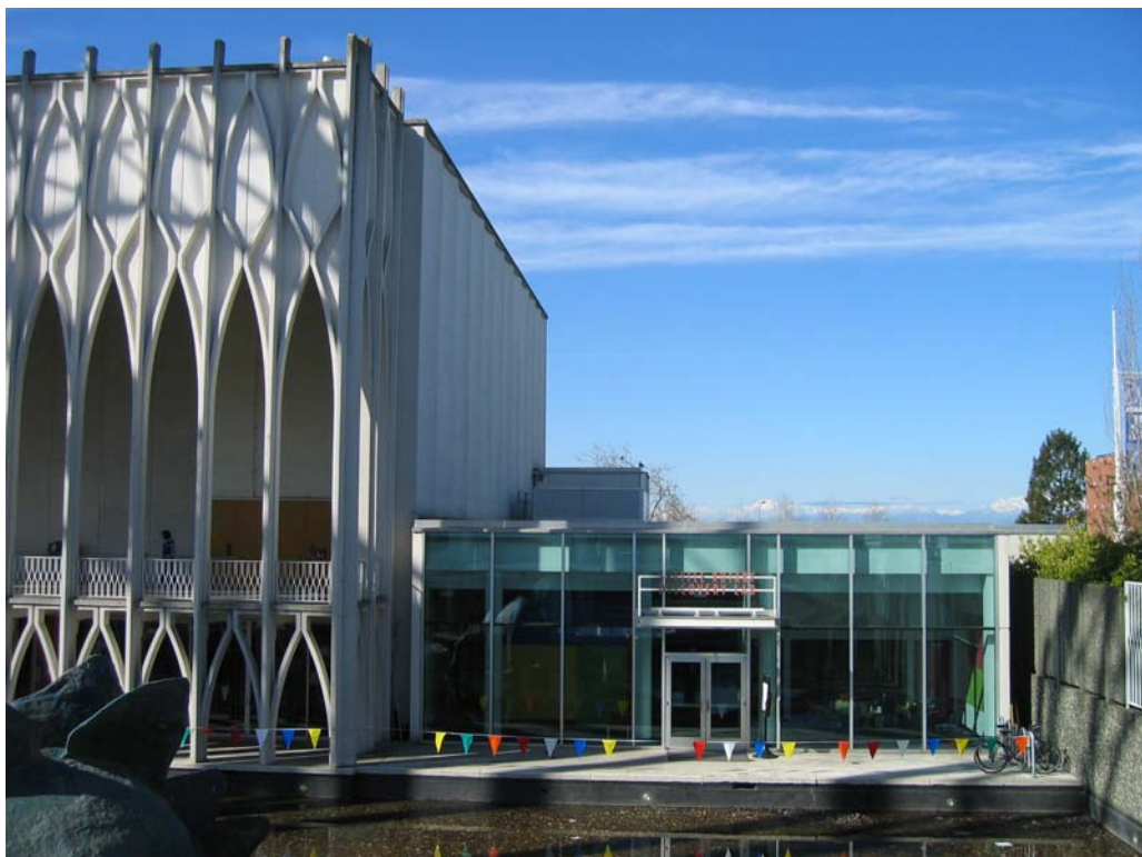
Figure 43 – Building 5 (1962: Building 1) on left, 1996 Discovery Labs addition on right (east elevation)
