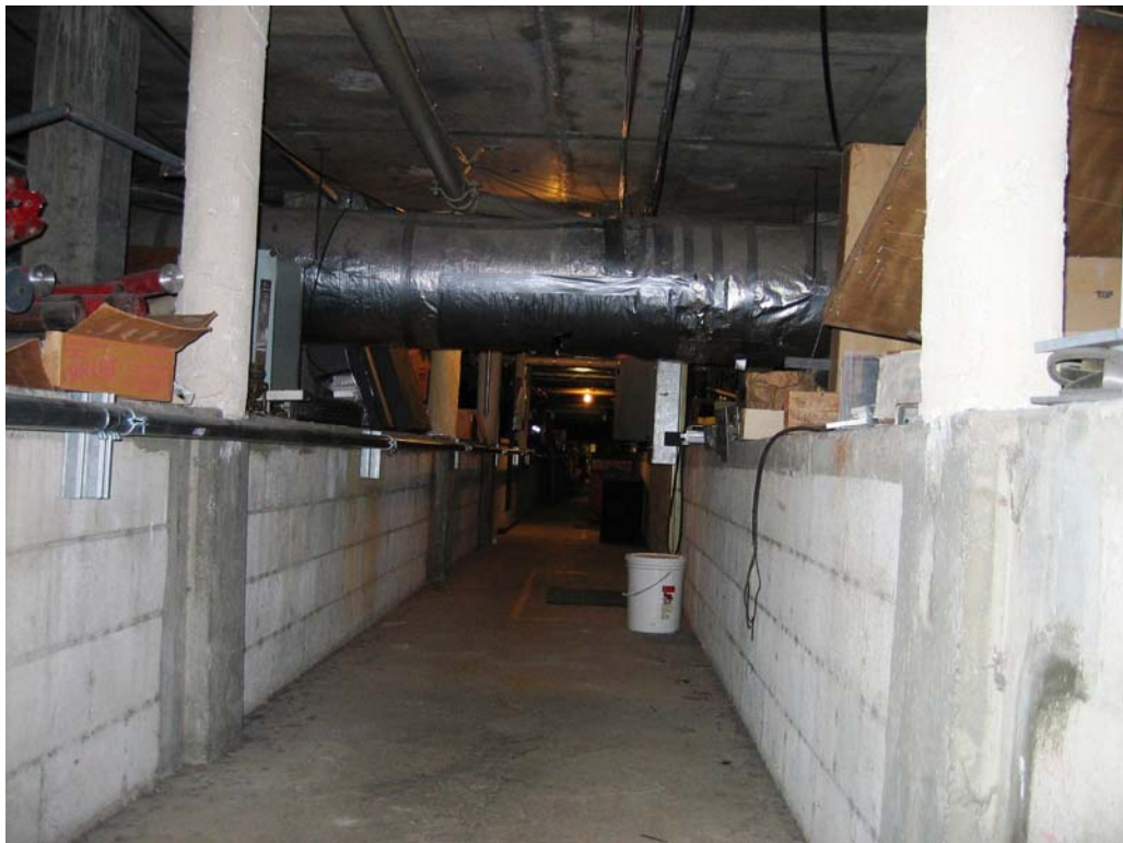
Figure 59 – Typical basement view under original 1962 buildings
