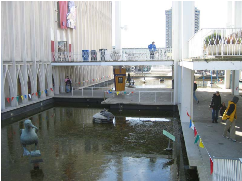
Figure 74 – 1962 walkways and railings
