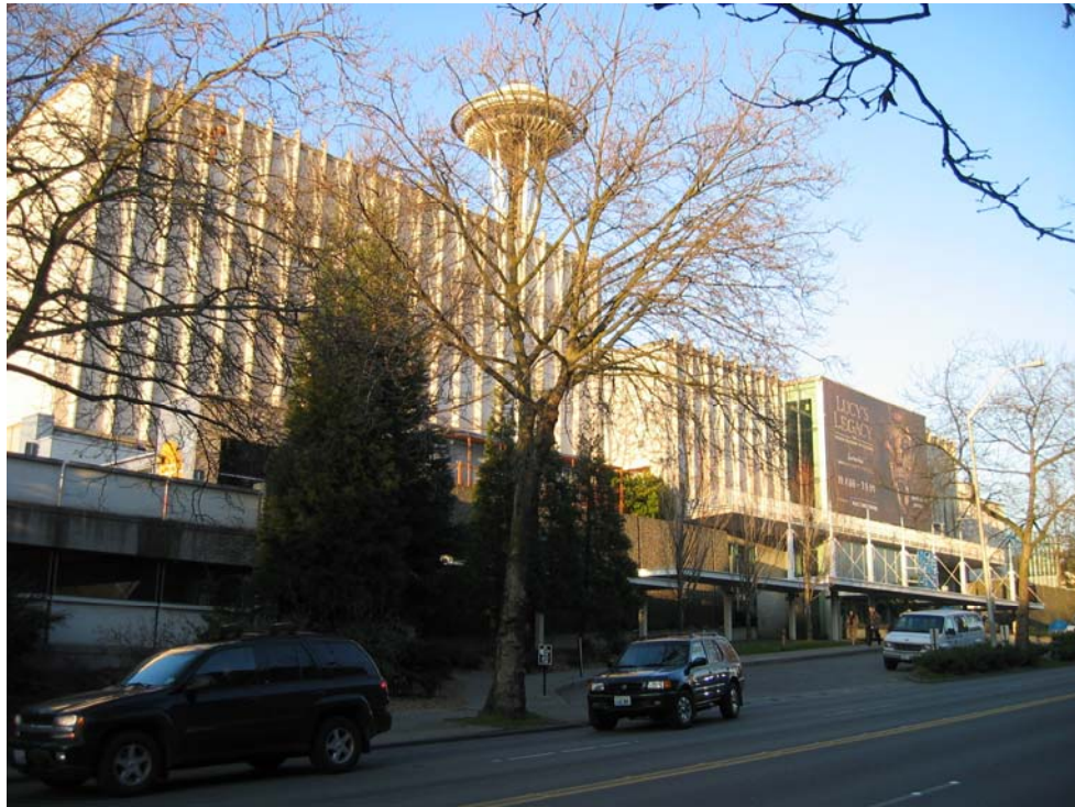
Figure 38 – Pacific Science Center south perimeter elevation showing additions to Building 3 (1962: Bldg R) on right
