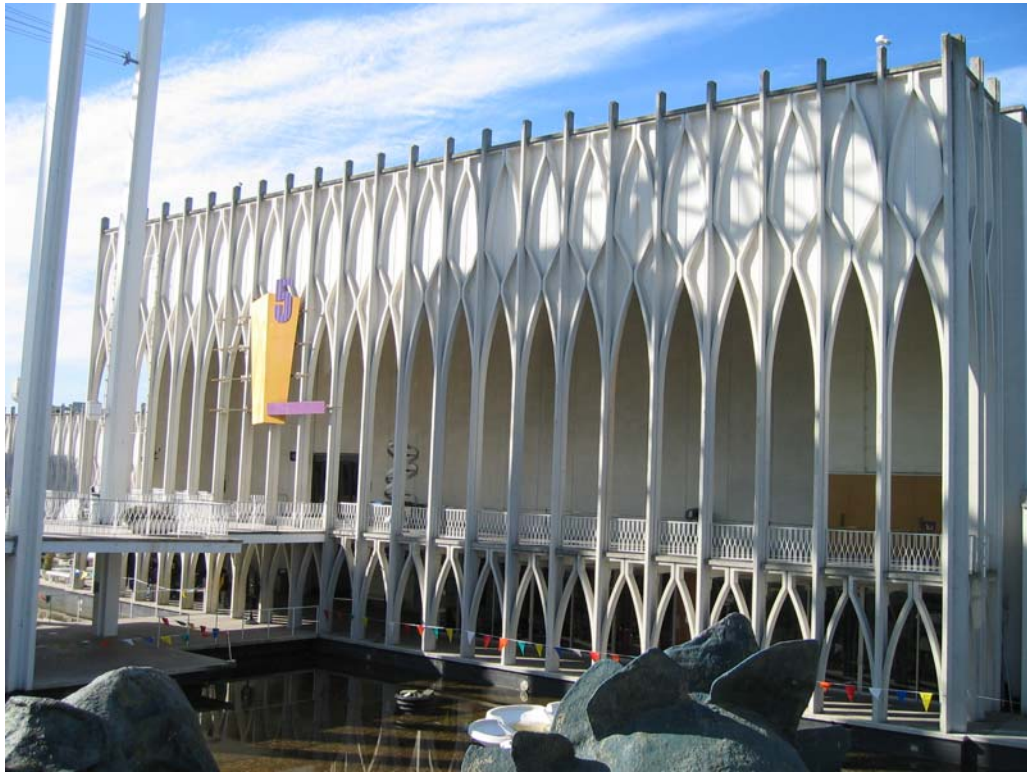
Figure 30 – Building 5 (1962: Building 1) east elevation, and walkways
