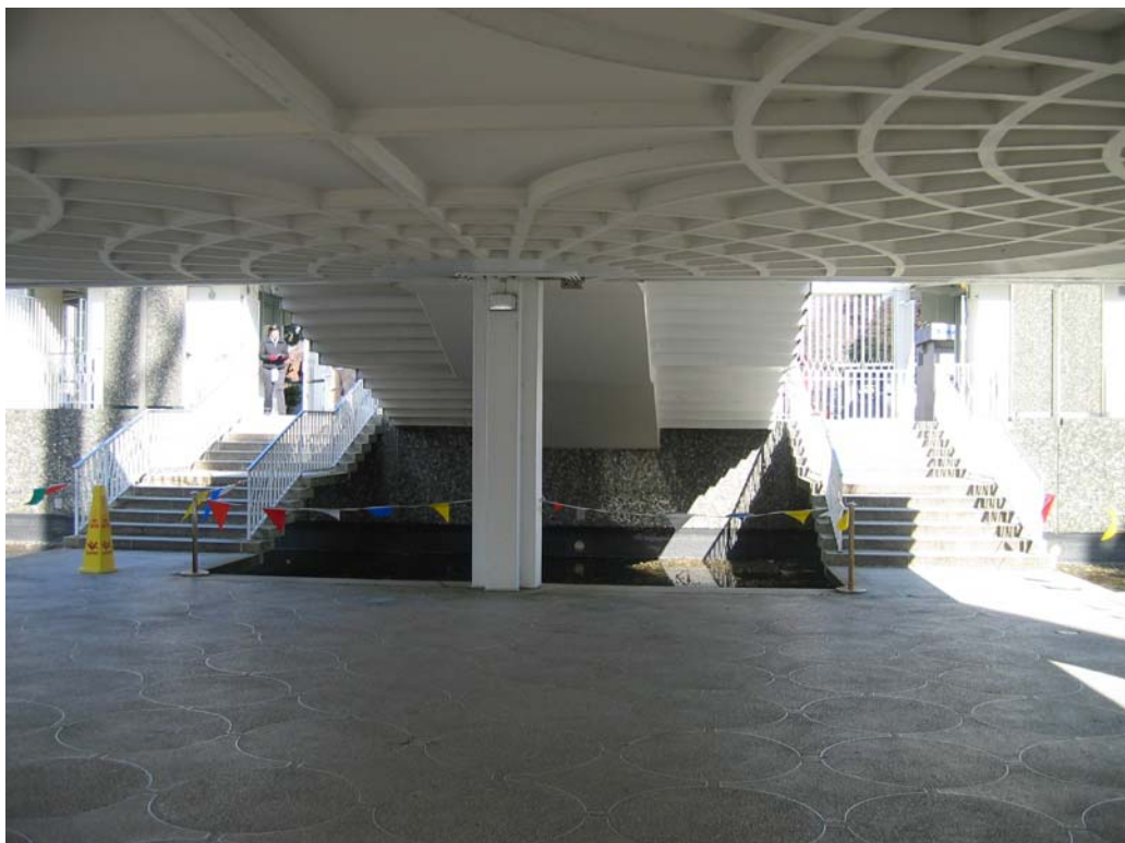
Figure 75 – 1962 underside of tower platform
