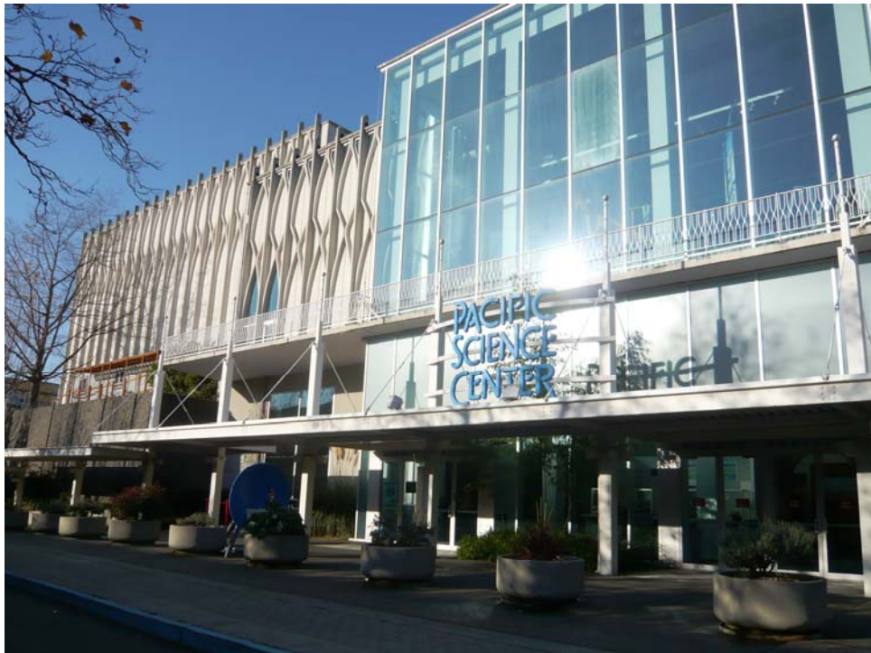
Figure 87 – South elevation of Building 4, Laser Dome, and Building 3 (left to right). The steel walkway canopy structure and large glazed bay dates to 1992-93 renovations to Building 3 (1962: Building R) to create a south entry at Denny Way. Railing and balcony at middle of picture is original to 1962 building.
