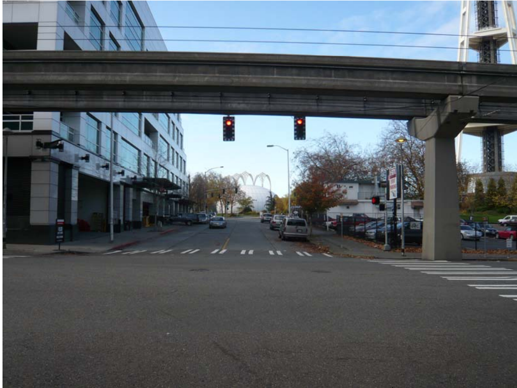
Figure 24 – Neighborhood context: view west from John Street and 5 th Avenue monorail tracks
