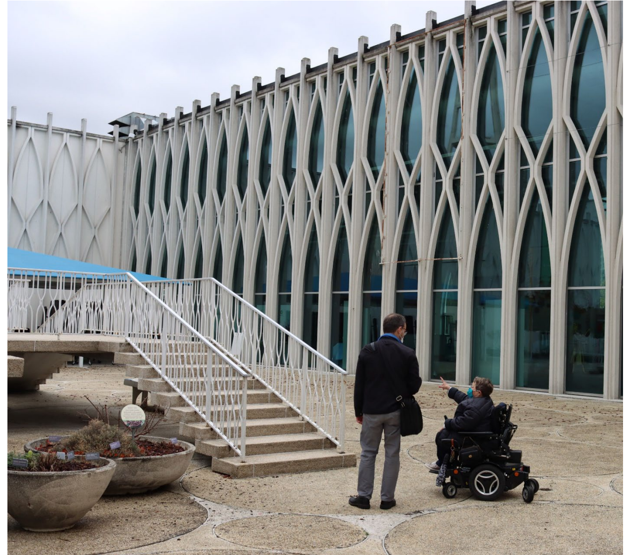
No Accessible Access to the Elevated Platform
