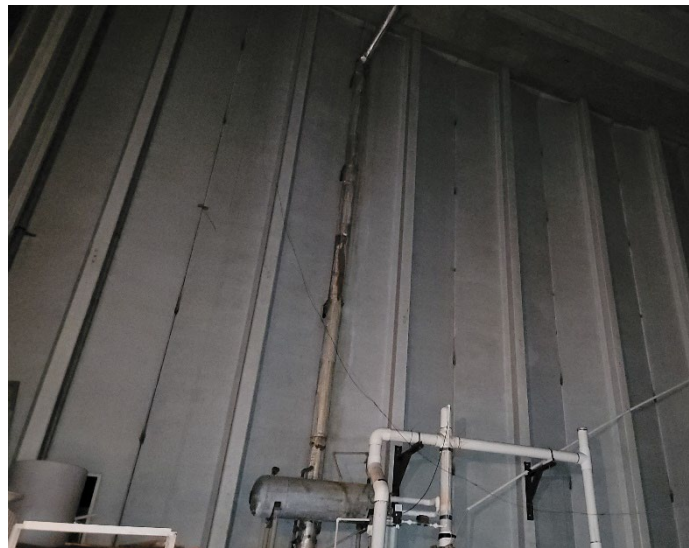
Interior View of Concrete Wall Panels
