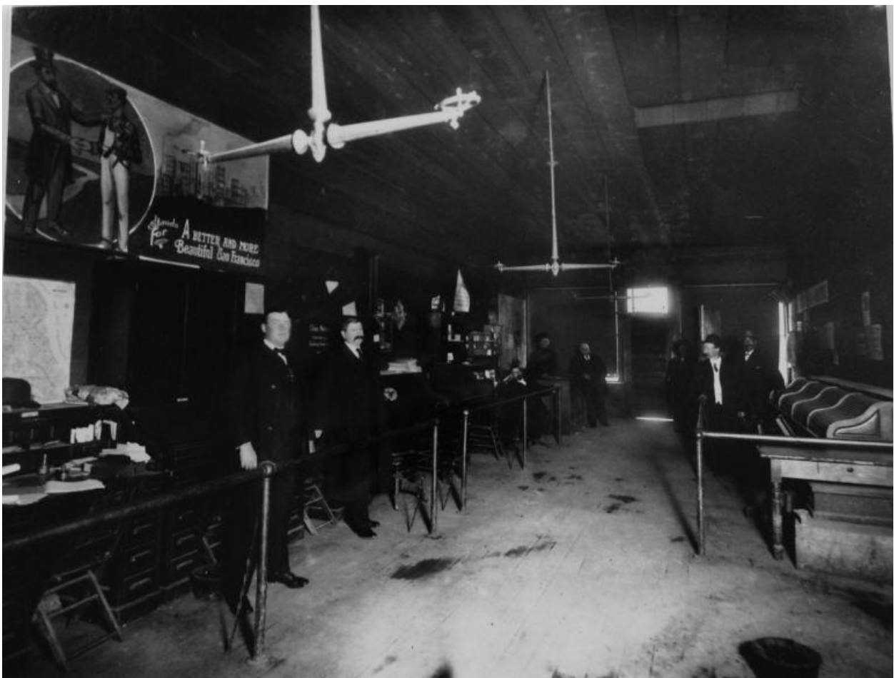
Figure 3 Building Trades Council- 14th and Guerrero interior, c. 1910.
