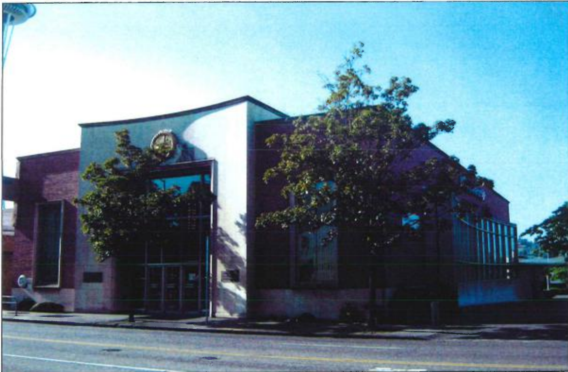
A similar view today, looking northwest toward the south and east primary facades of the building.
