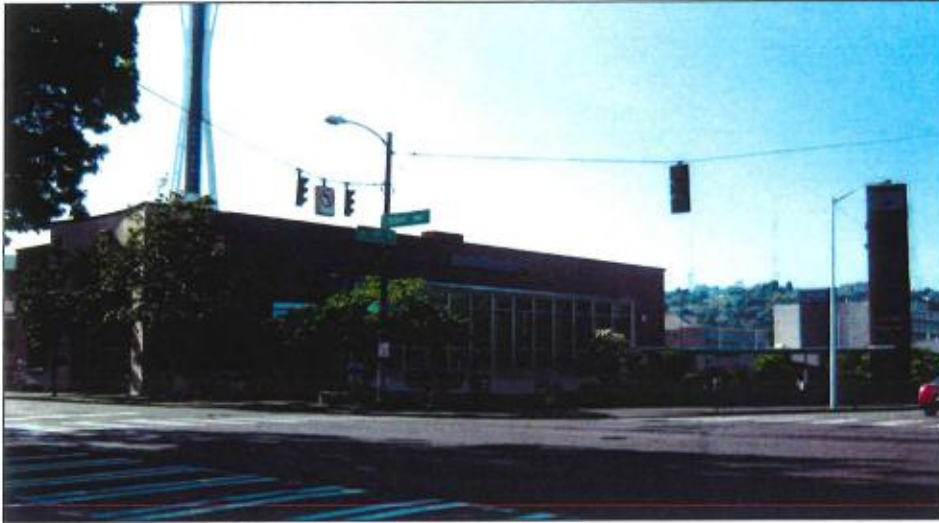
View looking northwest toward the building, showing the east facade and the relationship of the 50' tower to the building. Note the concrete marquee connecting these two elements.
