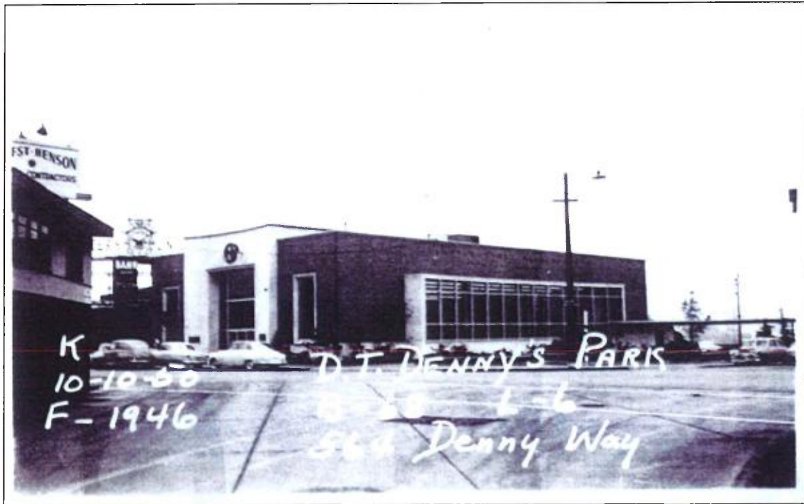
A tax record photo shows the bank building soon after it was completed. View looking northwest, October 19, 1950. (Puget Sound Regional Archives.)
